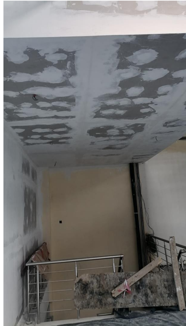
Gypsum Works - Ceiling
