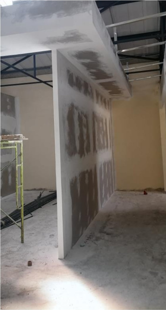
Gypsum Works - Partitions
