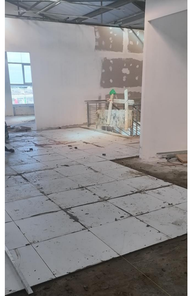
Floor works - Tiling
