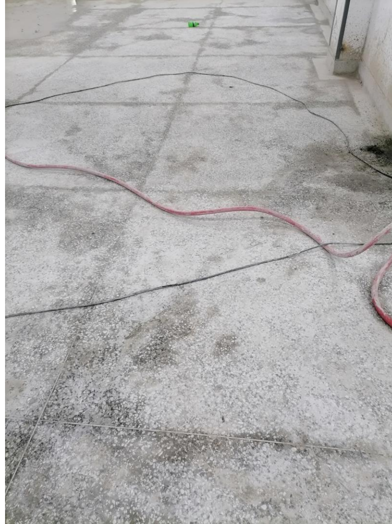
Floor works - Terrazzo
