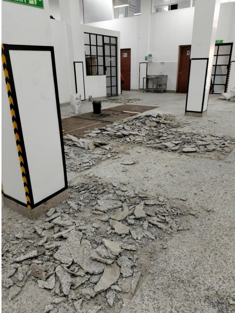
Floor works - Terrazzo
